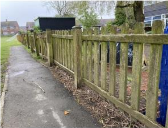
Fence repainting, ongoing
